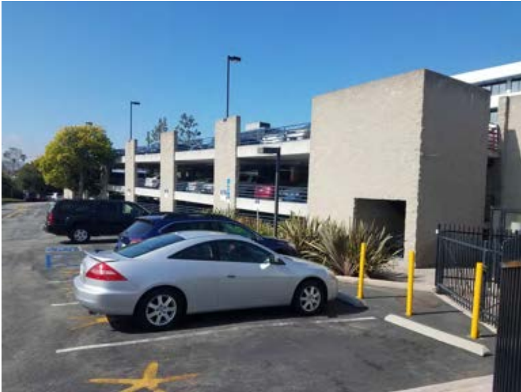
View of above-ground, four-level parking structure.
