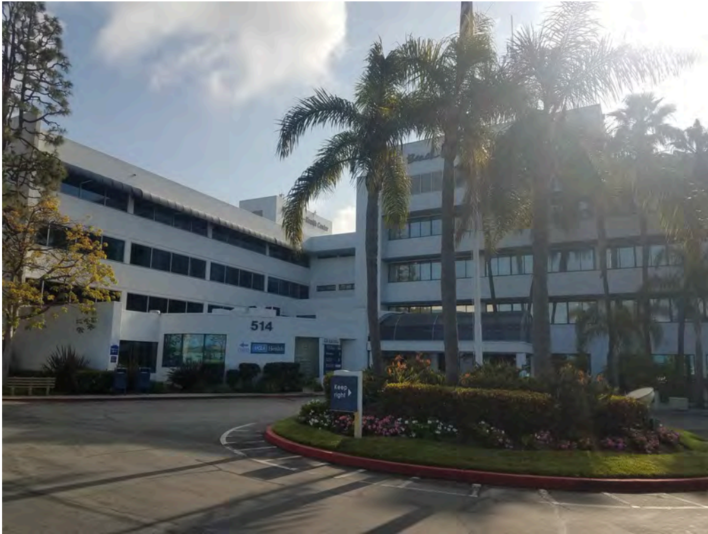
View of former hospital building/current medical office building (514 N. Prospect Ave.)
