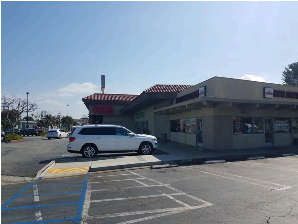
View of northwestern adjoining retail strip center (1202-1262 Beryl Street).
