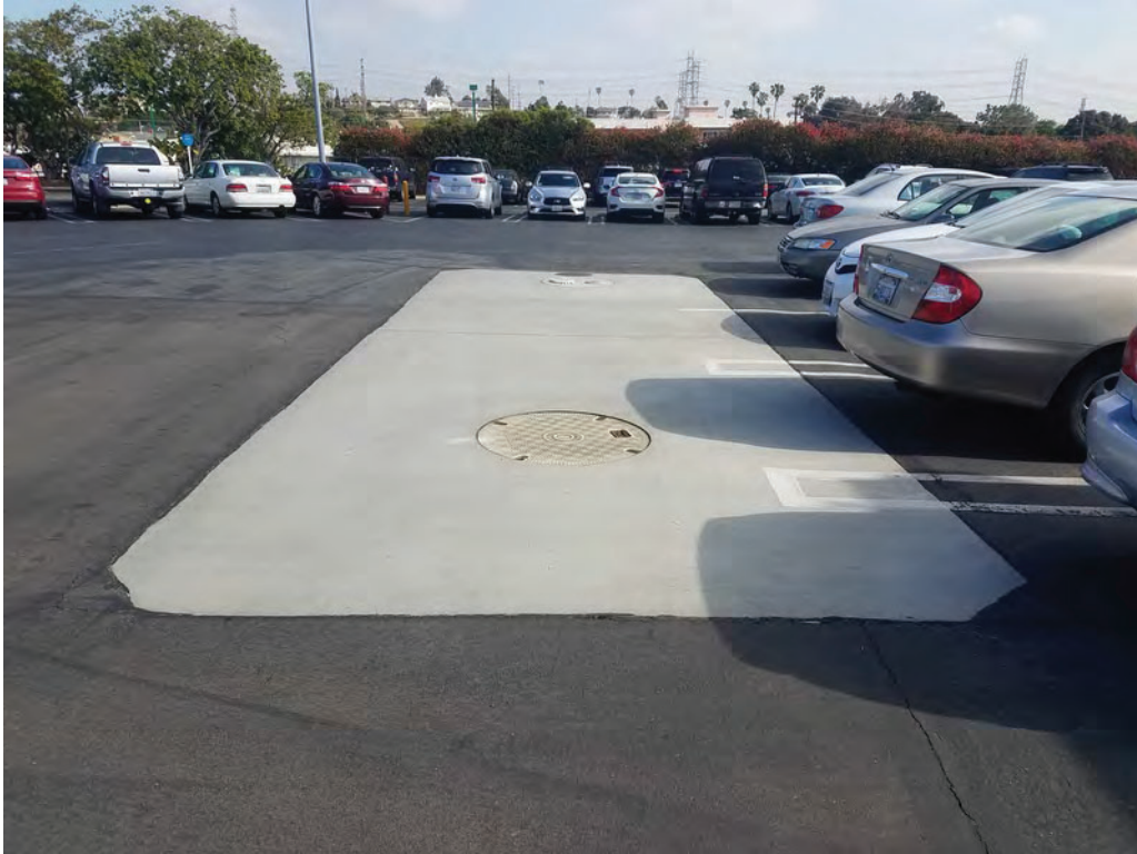
View of concrete patch and fill ports above the 10,000-gallon diesel fuel UST.
